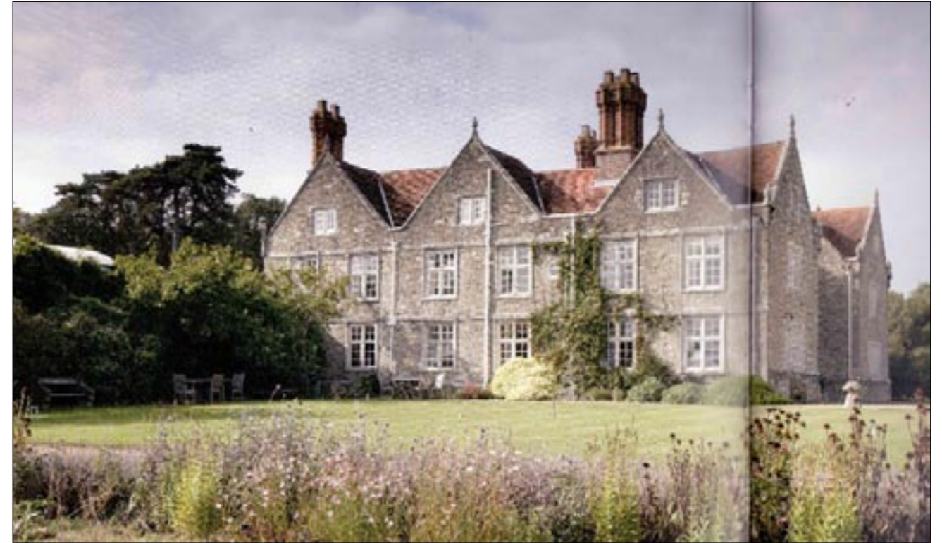
EXISTING SOUTH EAST FACADE WITH NO TERRACE AND OUTDOOR ACCESS
