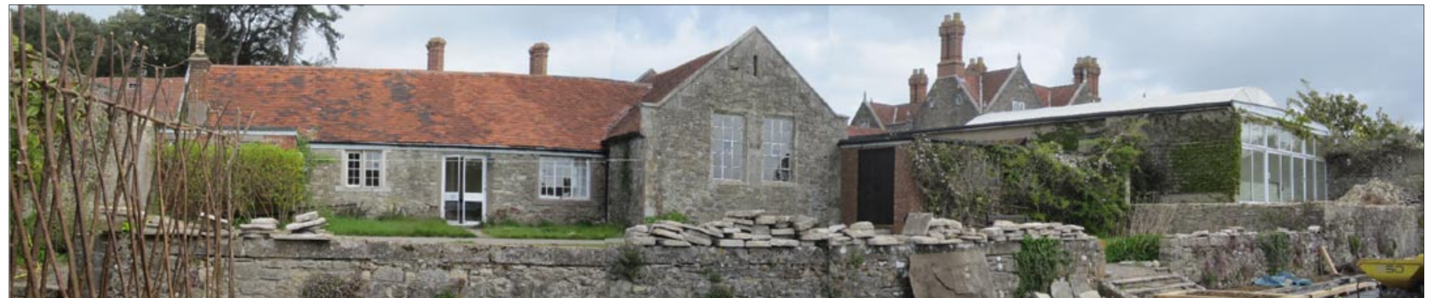
EXISTING COTTAGE, COACH HOUSE, CARPORT AND INDOOR SWIMMING POOL AS VIEWED FROM WALLED GARDEN WITH BARTON MANOR IN BACKGROUND
