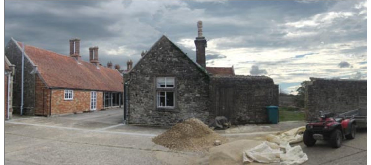
COTTAGE, ENTRY TO WALLED GARDEN AND BILLIARD ROOMS
