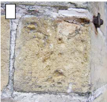
Images 1,2 & 3: Inclusions within fabric of brick.
