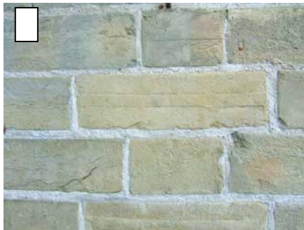
Images 1,2 & 3: Inclusions within fabric of brick.
