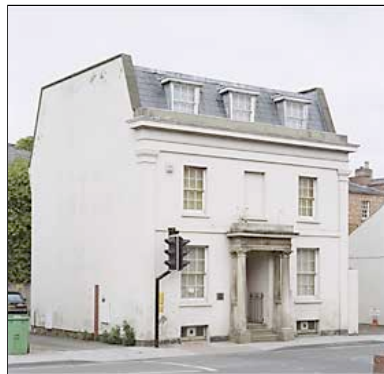
[Above] Another typical Georgian house in Cheltenham, showing an M-shaped roof with similar gable end to Farringford.
