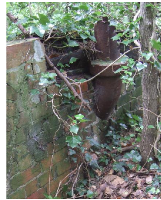
Girder (left) running off the end of the rear section into space, above the lower front section (centre). Flue outlet (right) for a stove.
