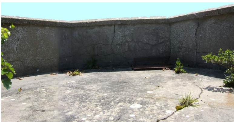
Lookout section showing hatch against W wall
