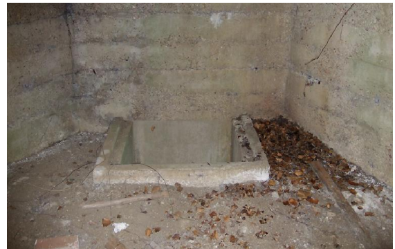
Internal entrance at base of gunner's section
