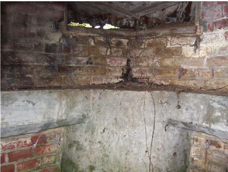
Gun platform with firing window above
