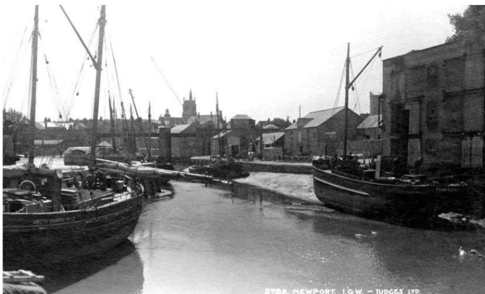
Figure 18 - Derrick and Model Stores, c. 1910
