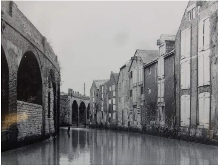
Figure 11 - 1970s view of the demolished Sea Street warehouses - the central three shown in Horatio Bennett's late C18 watercolour
