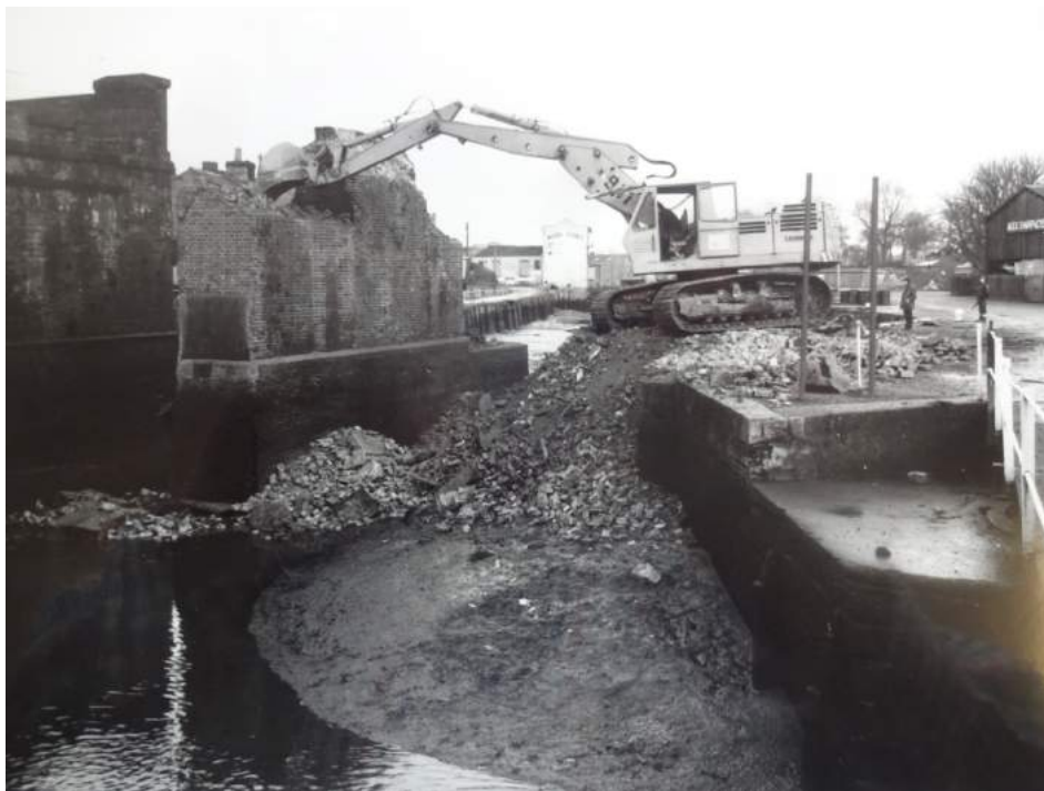
Figure 27 - Viaduct being demolished, c. 1973
